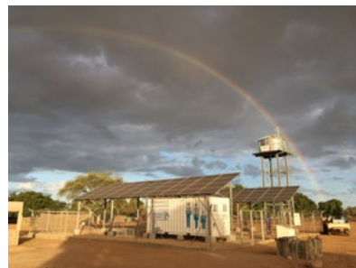
Solar powered brackish water treatment unit OSMOSUN® for community water production in Mozambique
